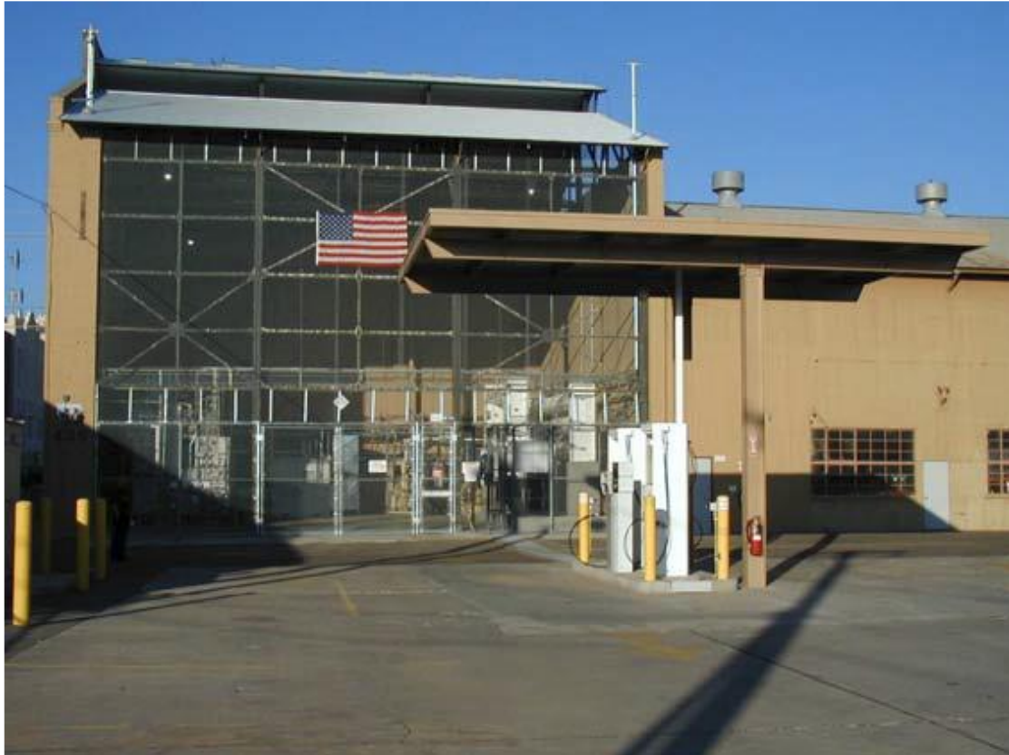
Figure 2. APS Hydrogen Pilot Plant, Phoenix, Arizona 1 .
